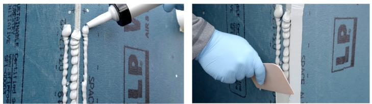
Apply a bead in the gap between corner panels and on both sides of the corner.Finish as above for panel seams. (Tip: A corner trowel may help.)
